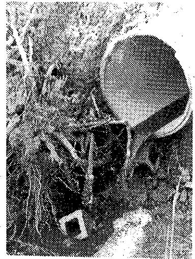
The drainpipe outlet
